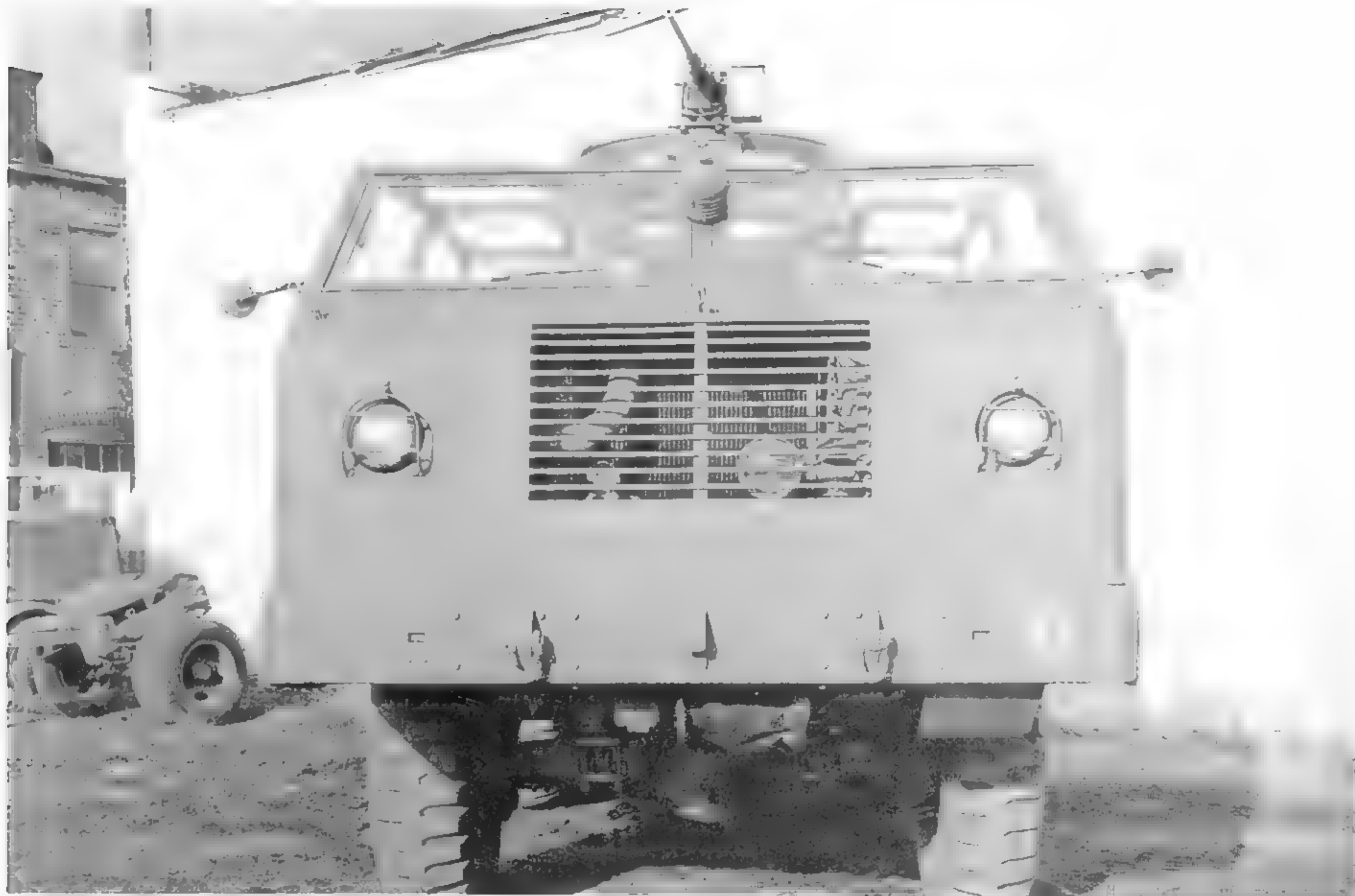
In November 1944, this soft-skinned M26A1 was photographed at the Engineering Standards Research Laboratory. Being some 10 tons lighter than its predecessor, the M26A1 had considerably better off-road performance and increased load-carrying capacity. (U.S. Army photo)
